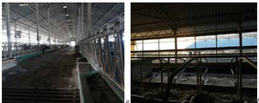
Figure 2. Lightweight premise frame for 600 milk cows: a) inside view of the premise from the side of feed table; b) boxes for cows rest
