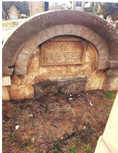
Fig. 3. General view of the crypts located in the Pirshahid cemetery (20th century)
