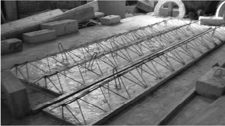
Figure 4. The view of the reinforced formwork floor slabs after their manufacture [8; 9]
