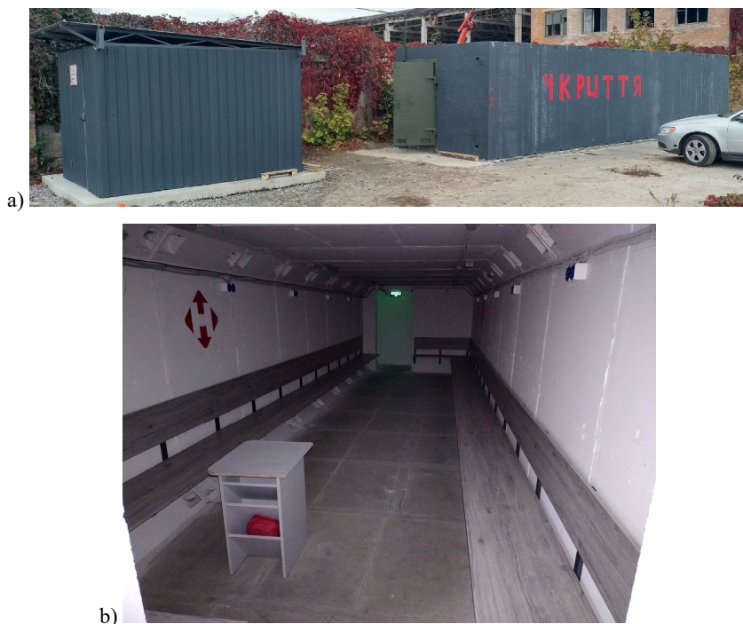
Figure 1. Mobile shelter installed near the Nova Poshta logistics center in Poltava: a) exterior view; b) interior organization
