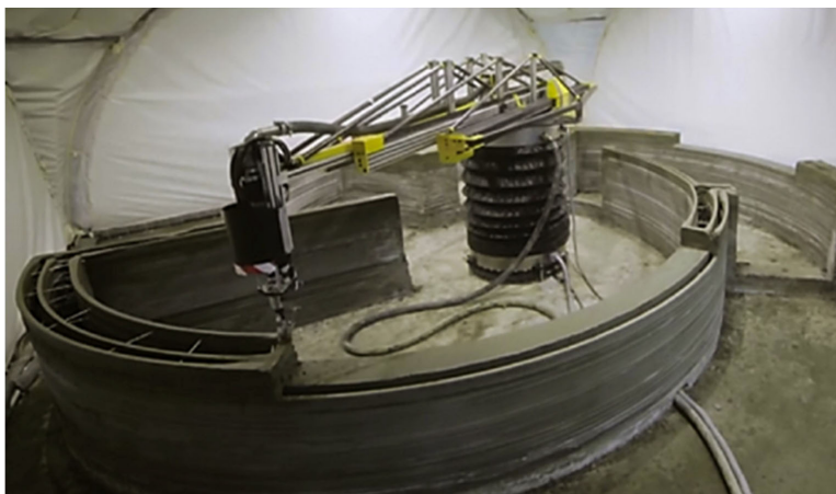
Figure 5. Construction of a shelter using 3D printing
