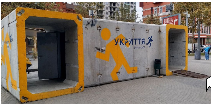
Figure 3. General view of a temporary protective structure at urban transport stops in Dnipro with an accessibility element for people with limited mobility
