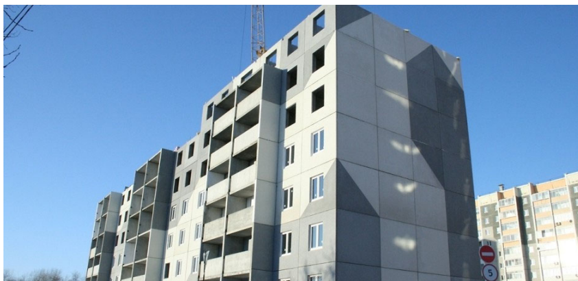
Figure 3.1 – General view of a typical large-panel building
