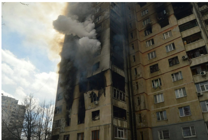
Figure 3.3 – Multi-storey building on Pivchnaya Saltivka in April 2022 [50]
