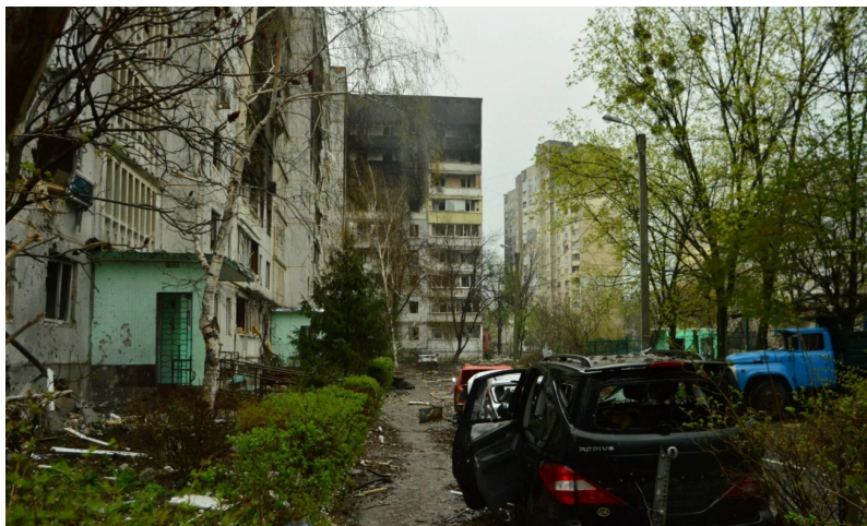
Figure 3.4 – Multi-storey building on Pivchnaya Saltivka in April 2022 [50]
