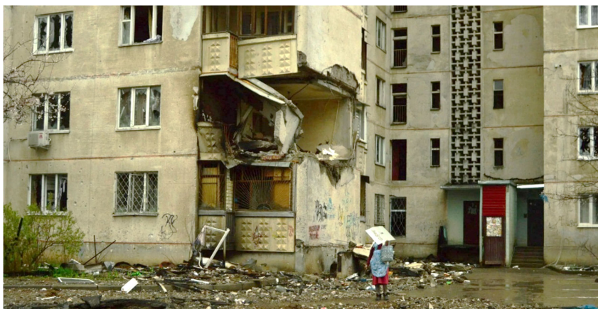
Figure 3.5 – Multi-storey building on Pivchnaya Saltivka in April 2022 [50]
