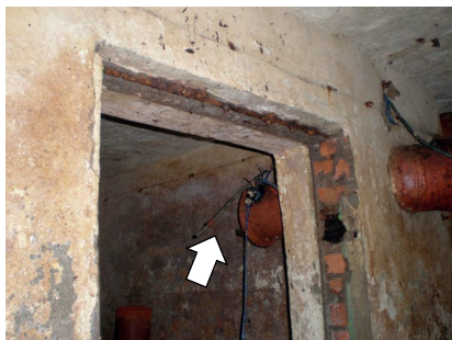
Figure 3.5. Partially dismantled ventilation system of the premises
