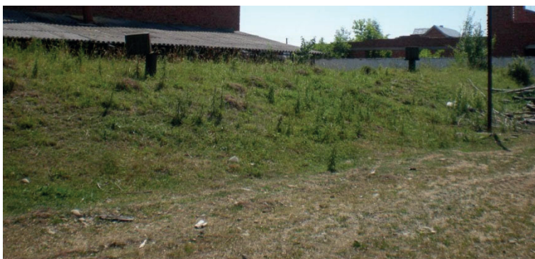
Figure 3.11. General condition of the territory adjacent to the bomb shelter
