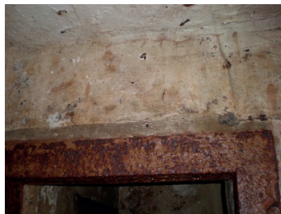
Figure 3.7. Corrosion damage of steel door frame elements
