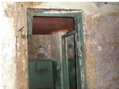
Figure 3.9. General interior view of sanitary facilities
