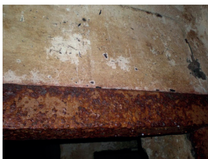
Figure 3.7. Corrosion damage of steel door frame elements
